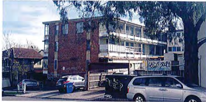
Figure 2.05: Site 2 - Carlisle Street facade
