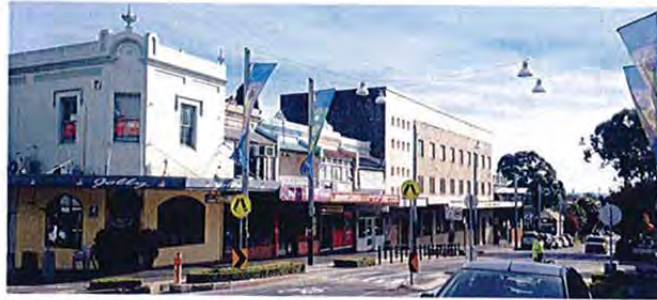
Figure 2.01: Site 2 - 168 Norton Street - Harold Hawkins Court
